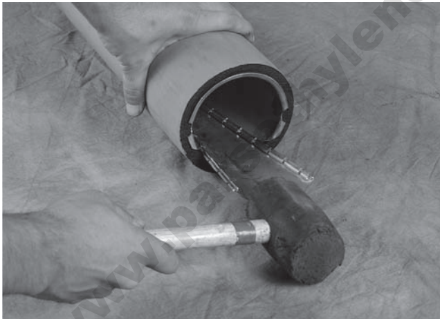
Figure 12 Install Split Ring Stiffener in PE Pipe
