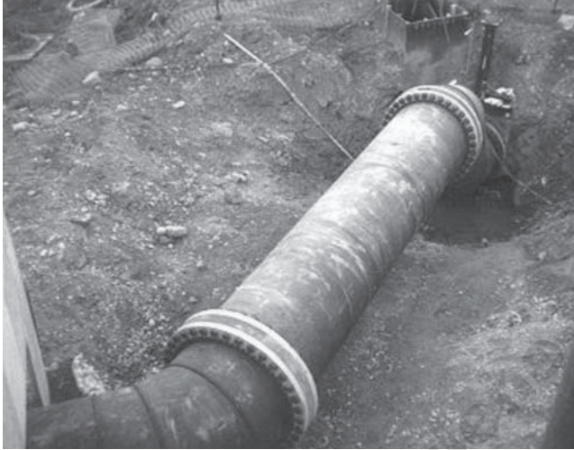
Figure 13 Flange Adapter Assembly
