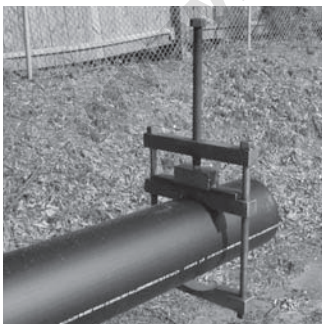
Figure 15 Mechanical Re-Rounding Clamp Installed
