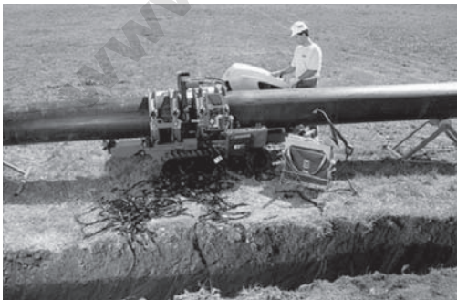
Figure 1 Above Ground Repair with Fusion Machine
