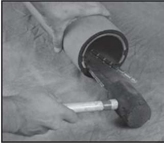
Figure 19 Install Split Ring Stiffener in PE pipe
