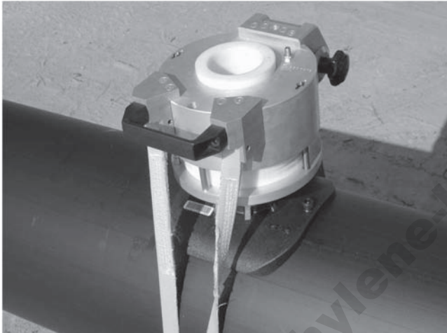
Figure 4 Electrofusion Patch Repair
