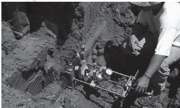
Figure 3 Saddle Fusion Repair
