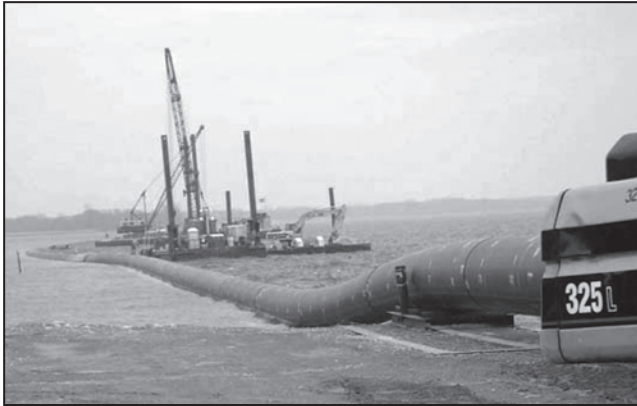
Figure 5 Unballasted PE Pipeline Being Floated Out to Marine Construction Barge Where Ballast Weights are Installed
