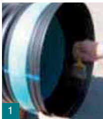
1 Apply lubricant to the inside of the belling.
